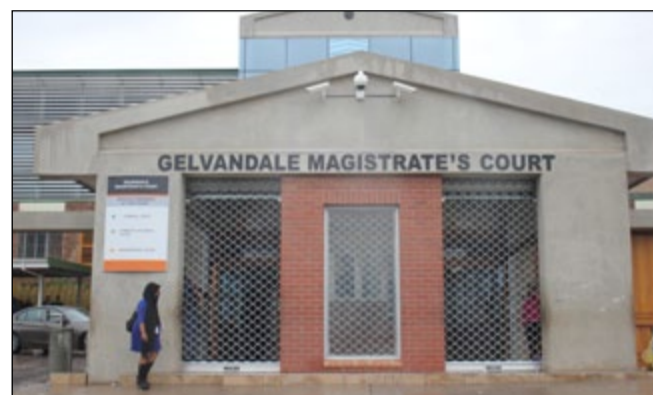
The newly-renovated Gelvandale Magistrates' Court
