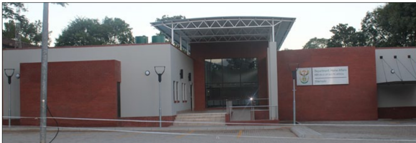
The Makhado Home Affairs service centre in Limpopo, handed over to Home Affairs by Public Works Minister Mr TW Nxesi
