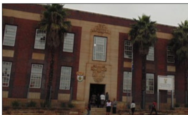
The revamped Pietermaritzburg Magistrates' Court - Annex Building
