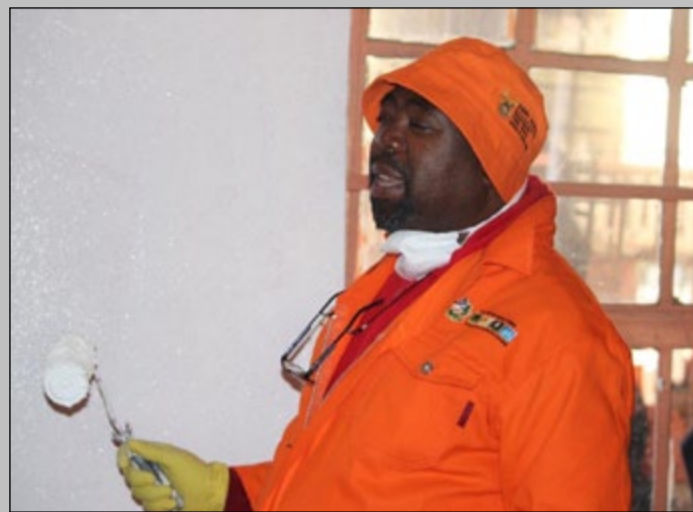
Public Works Minister TW Nxesi repainting the walls of a school in Atteridgeville
