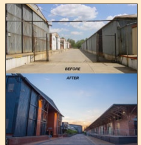
Before and After the restoration of the hangar & platform type building
