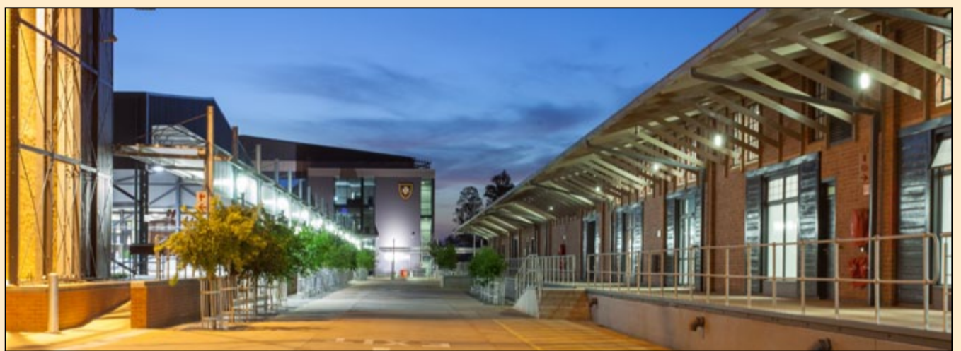
Restored heritage buildings on both sides of the existing internal road with Building A entrance in the background
