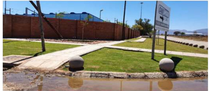
Figure 9: Lebowakgomo SAPS, Juncture between South & East exterior. Photo by: Lunga Sithole.
