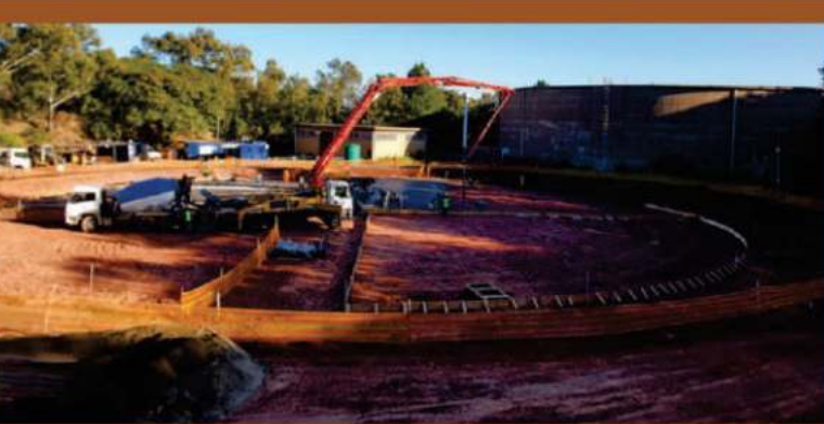
The remaining four government head offices to be constructed in the precinct includes the Department of Social Development and its agencies, the South African Social Security Agency and the National Development Agency, the Department of Higher Education and Training, the Department of Home Affairs and the Department of Correctional Services and Constitutional Development.
