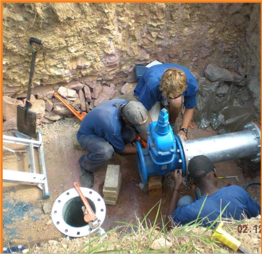
Pipe repair underway – another initiative by Public Works to save water
