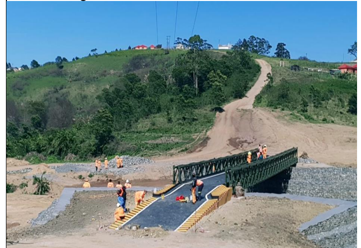
Cwaka during construction
