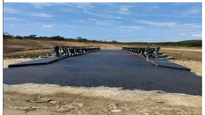
Mqothwane | During construction
