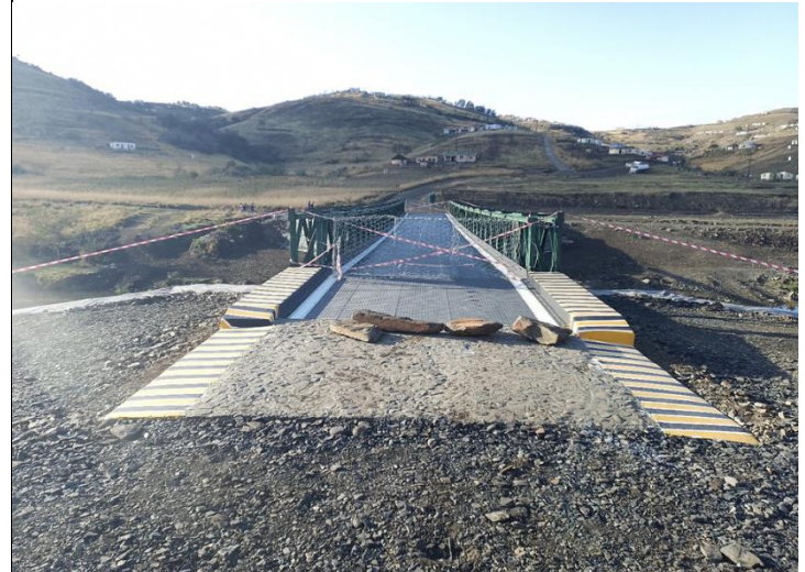
Mdlankala – DURING CONSTRUCTION
