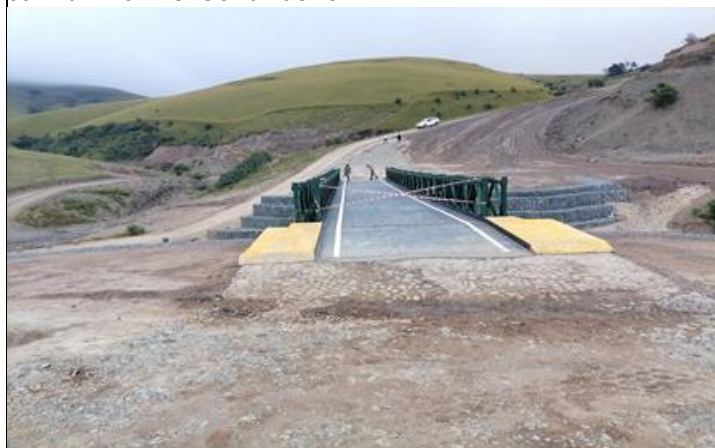
SUNRISE- DURING CONSTRUCTION
