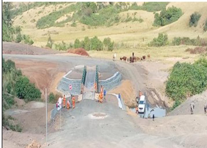
NTLENGA – DURING CONSTRUCTION
