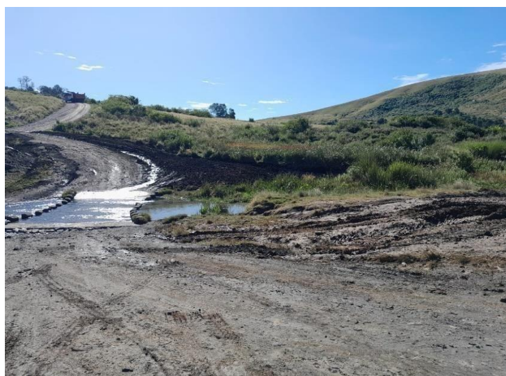
NTLENGA – BEFORE CONSTRUCTION
