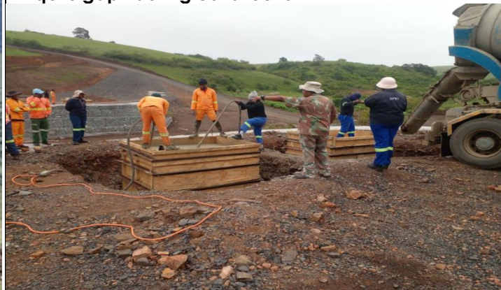
Mnqezu gap1 during construction
