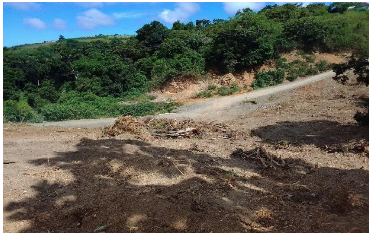
Dedeni before construction
