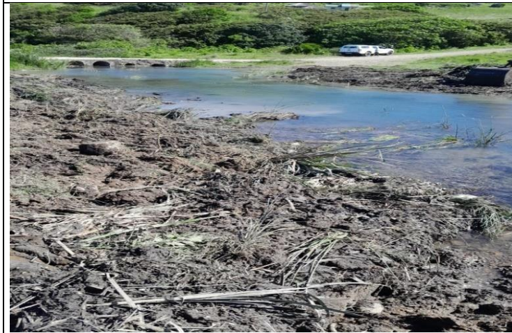
Mbotyi Before Construction
