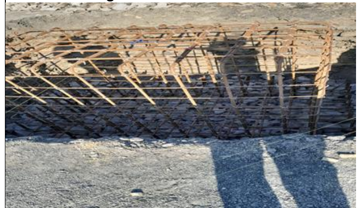
Mdwaka During construction
