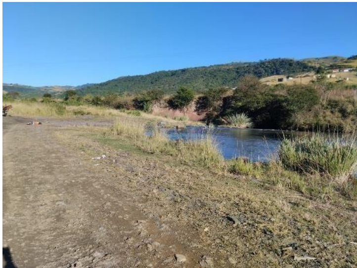
Mdlankala – BEFORE CONSTRUCTION
