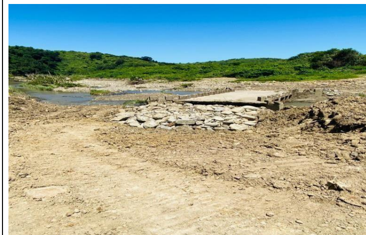
Rhebu Before Construction
