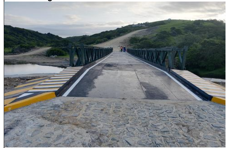
Rhebu During Construction
