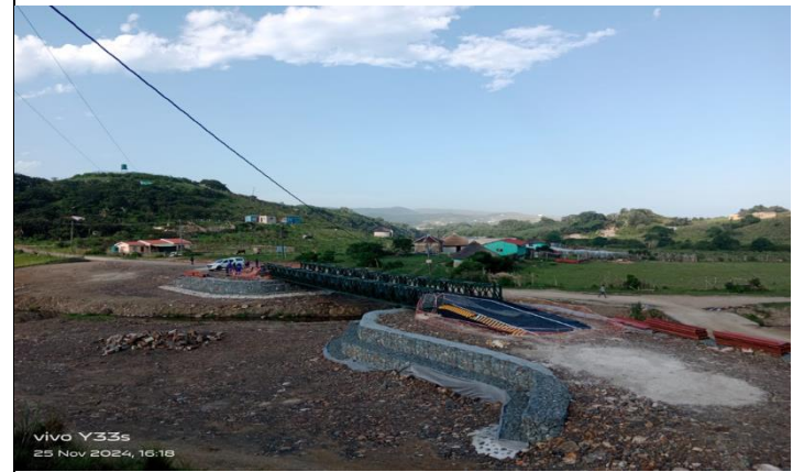
Mbotyi during construction
