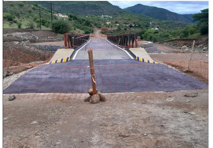
Dambeni During construction
