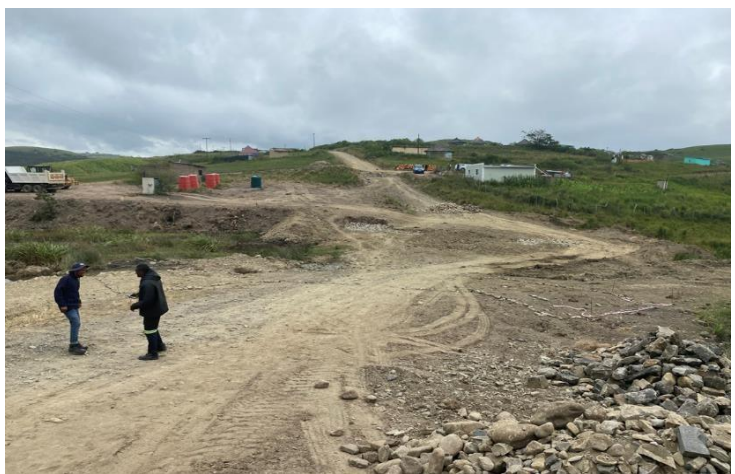
zixambuzi before construction
