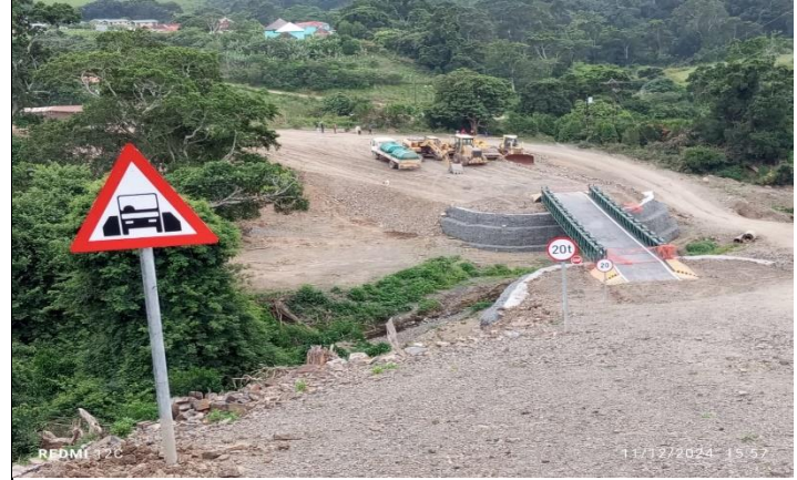
Dedeni during construction
