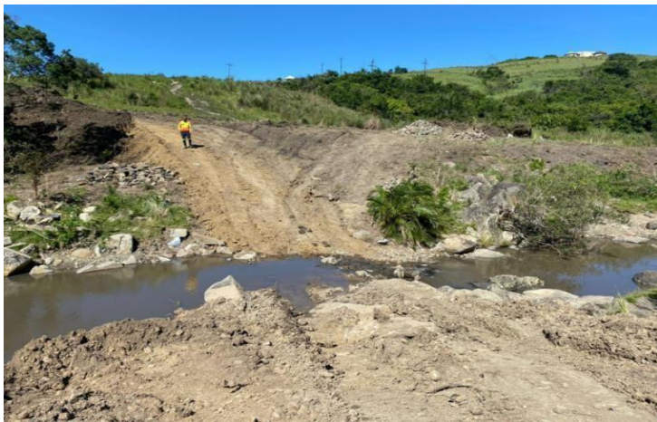
Mdwaka Before Construction
