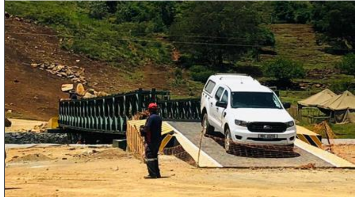
Mfundisweni | During construction
