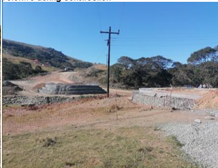
Folokwe during construction
