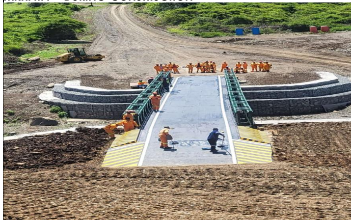
MKHATA – DURING CONSTRUCTION
