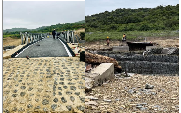
Mneno during construction
