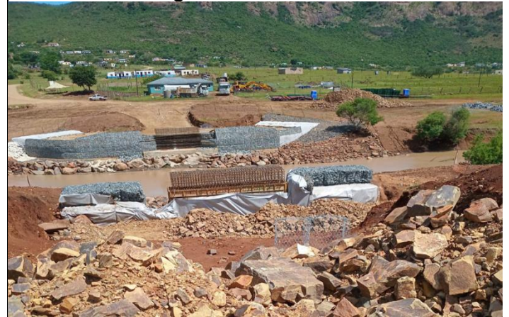
Emaxasibeni during construction
