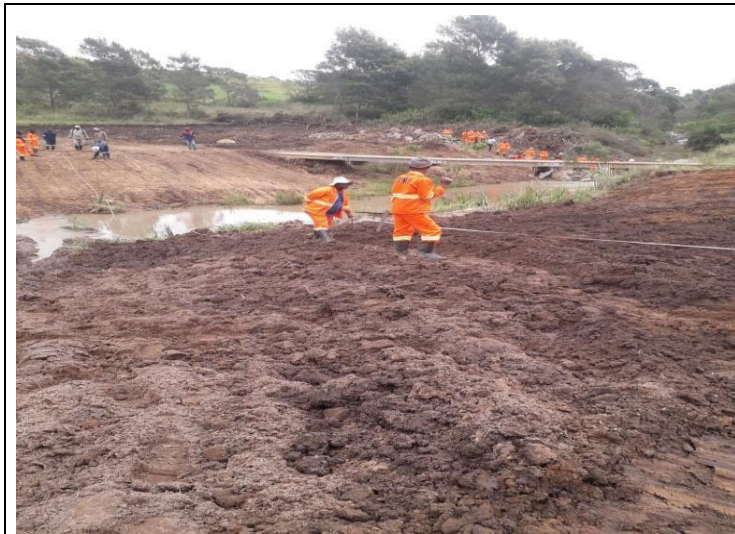
Cwaka Before Construction
