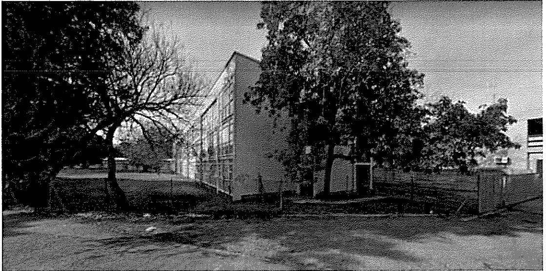
Figure 3: Site Photo of the 15 Flats
