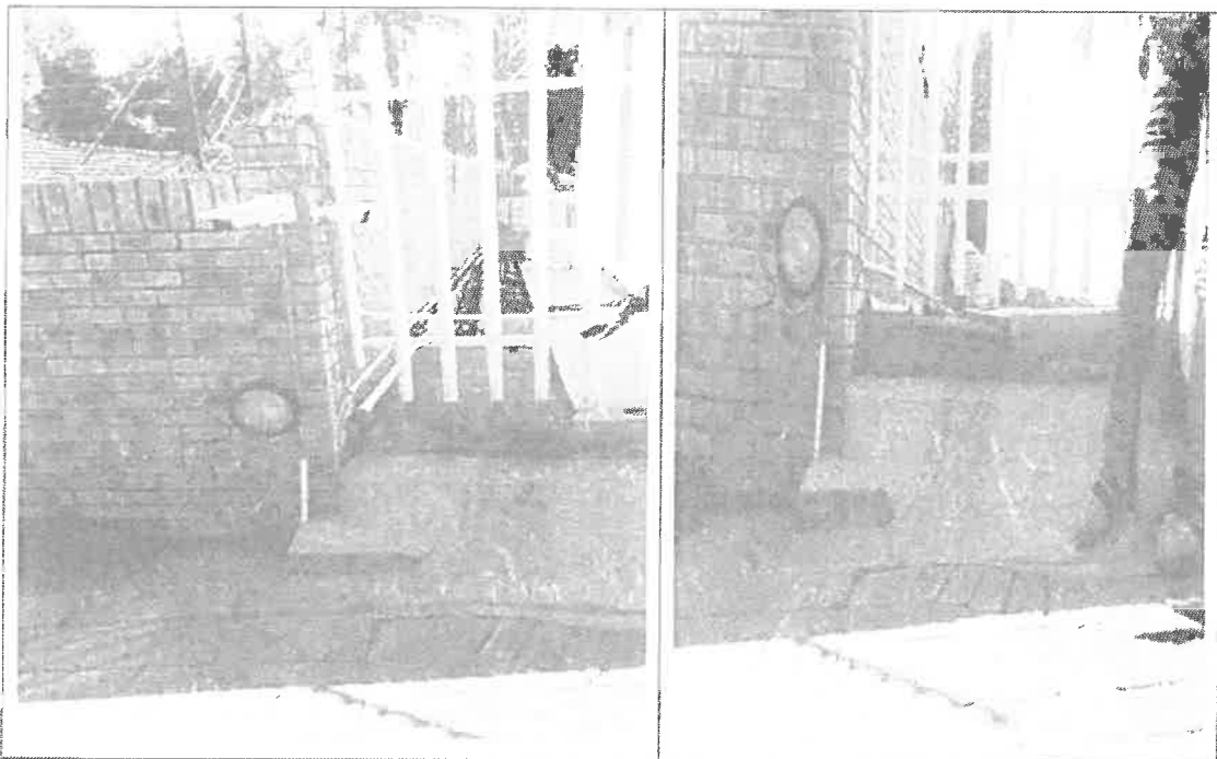
Figure 6: Surface bed and stairs
