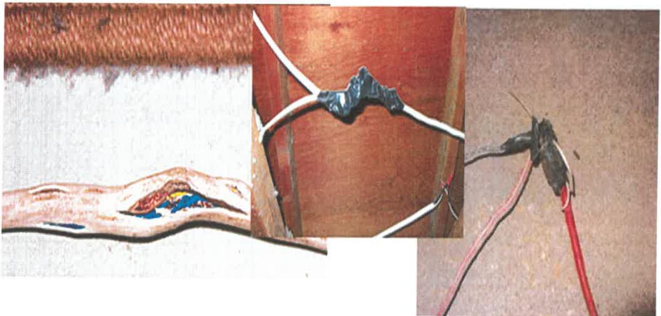
No joints are allowed on electric extensions cords. DB boards must have a COC certificate. We don't want to see any exposed wires like we see in the photo.
