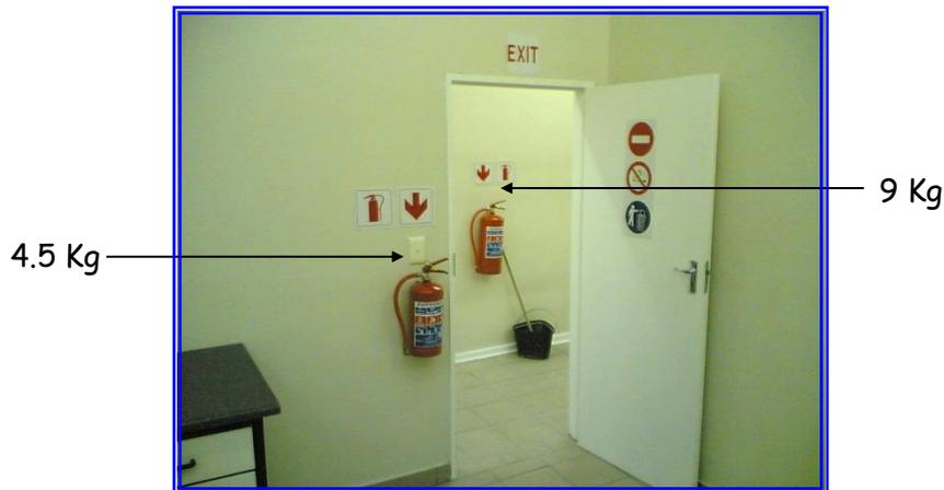
2. One (1) 9 Kg Dry Powder Fire Extinguisher shall be supplied and installed in the passage/area, wall mounted, outside of the Forensic Laboratory
