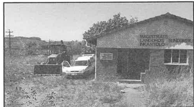
Plate 5: Existing single storey Magistrate Court building located on the site.
