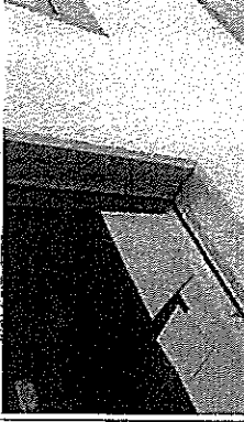
GLAZING: Glazing bead to Aluminum frame
