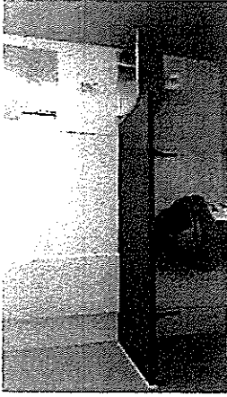
DISTRIBUTION BOX: Fully independent DB Box for SASSA All switches independently labelled Lockable and intruder proof
