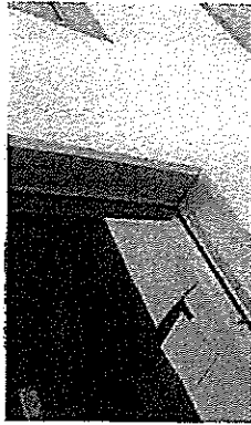
GLAZING: Glazing bead to Aluminum frame
