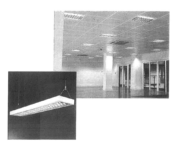
Lighting intensity to be a minimum 300 Lux on offices and 500 lux in public areas. To underside of ceiling fit 1200 flush recessed fluorescent light fitting with prismatic acrylic cover.
