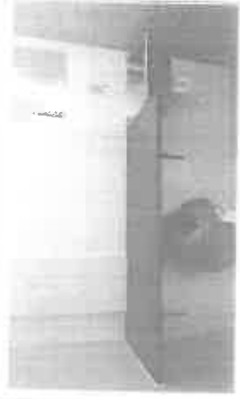
DISTRIBUTION BOX: Fully independent DB Box for SASSA All switches independently labelled Lockable and intruder proof
