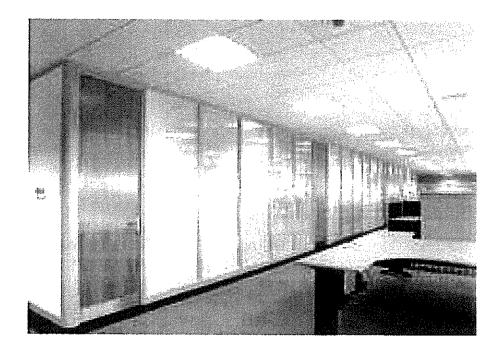
All doors are to be 0.813  $\times$  2032 x44mm flush laminated doors hung in standard steel door linings and fitted with two mortice locks with satin chrome plated handles. Steel door linings to be painted high gloss enamel paint C3-7. Doors to be painted eggshell enamel paint B20-7
