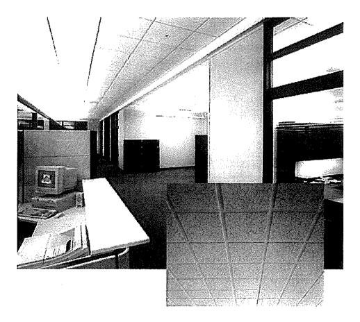
Ceilings can either be plastered concrete or gypsum plaster-board or suspended ceilings. All plastered or board ceilings to be painted with white PVA paint. Suspended ceilings are always designed at a height of 2.7 m from the finished floor which is a mandatory standard for all branches. Note: Deviation to a lower height of 2,4 m (absolute minimum) may only be considered in extreme circumstances.
