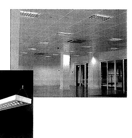
Lighting intensity to be a minimum 300 Lux on offices and 500 Lux in public areas. To underside of ceiling fit 1 200 flush recessed fluorescent light fittings with prismatic acrylic cover.
