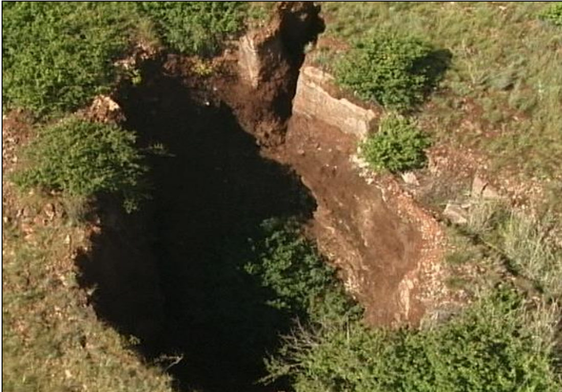
PLATE 1: Typical sinkhole (50m deep)
