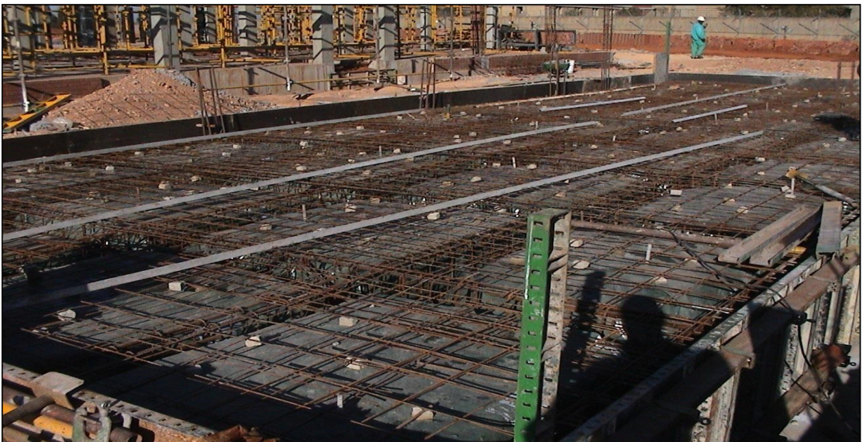
Plate: Typical reinforced raft foundation
