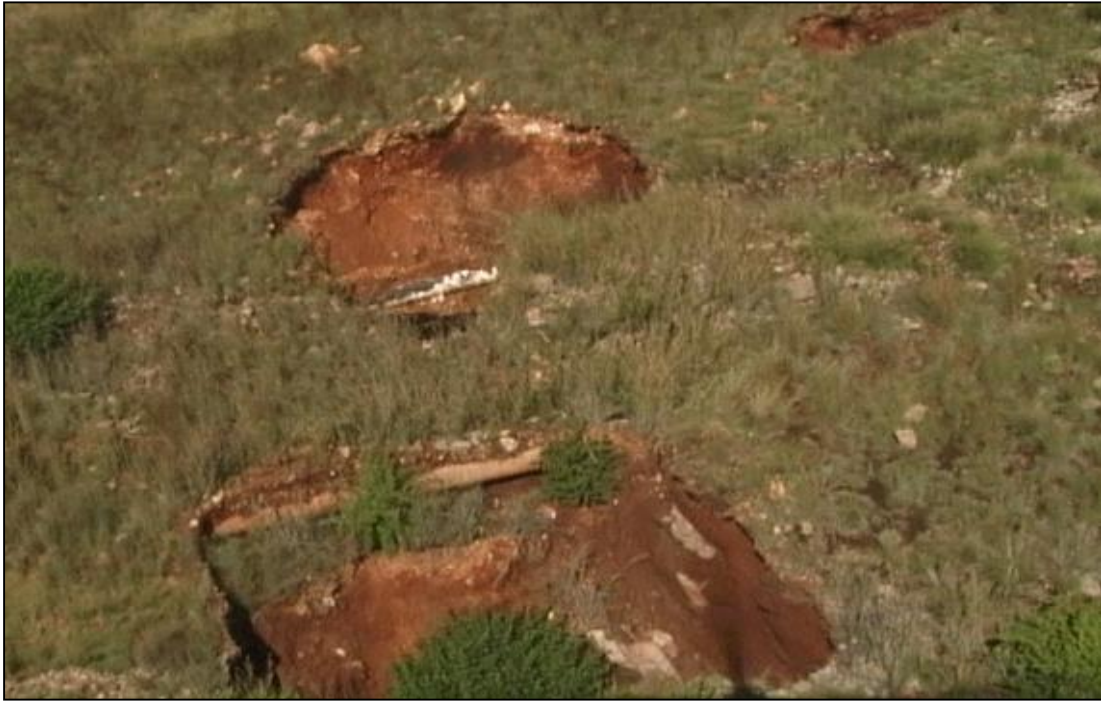
PLATE 5: Sinkhole as result of leaking water mains
