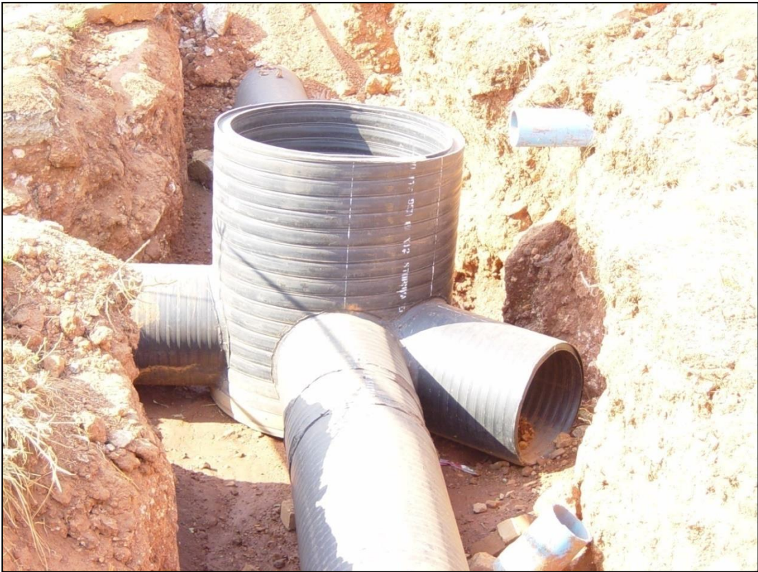
HDPE STORMWATER MANHOLE OF STRUCTURED WALL HDPE PIPE (SIDE VIEW)
