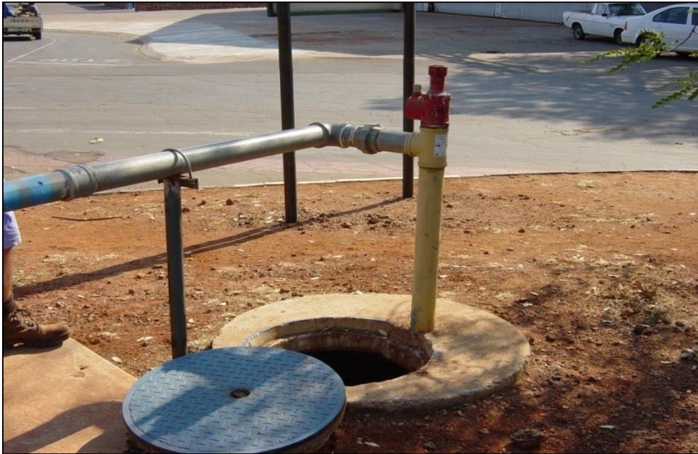
TYPICAL SURFACE MOUNTED WATER INSTALLATION
