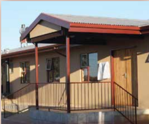
Newly built MYRA primary school outside Taung in North West
