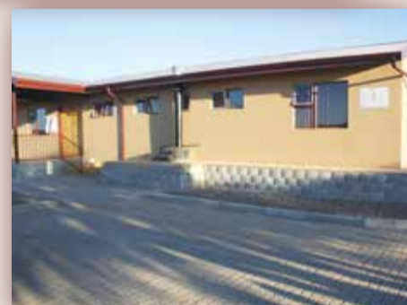
Myra Primary school fitted with the new toilet system and water harvesting tank
