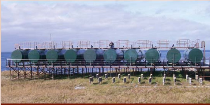
Fuel storage tanks at the island
