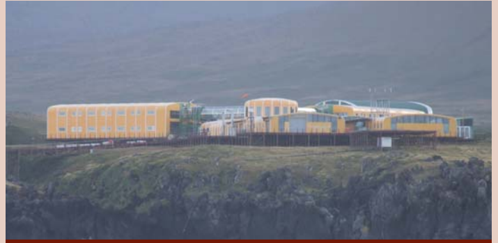
The completed base as seen from the ship anchored in the rough seas
