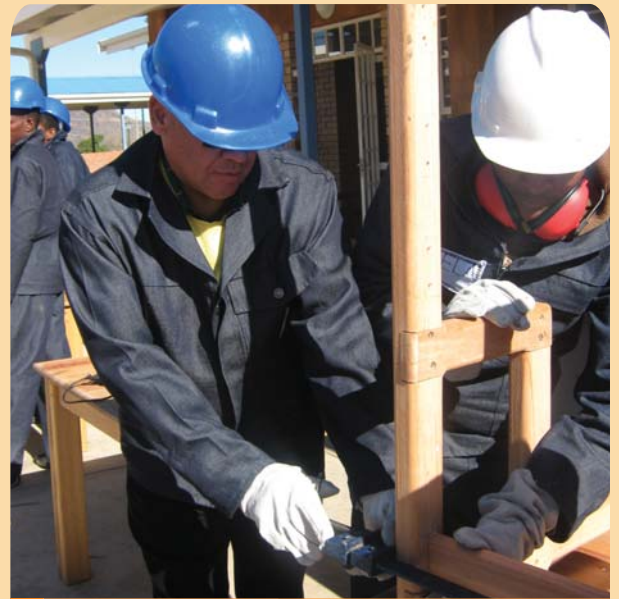
Minister Doidge hard at work assembling desks at Nolitha Special School
