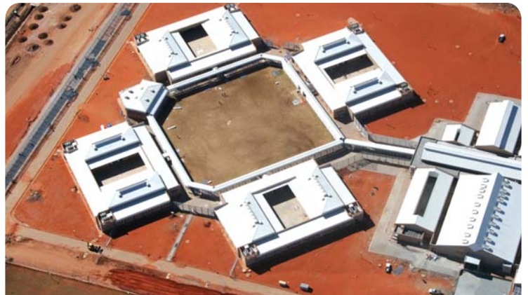
Kimberley's New Correctional Facility Aerial View
