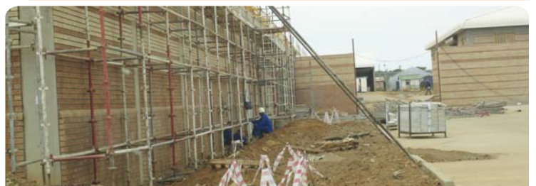
Kimberley's New Correctional Facility under construction
