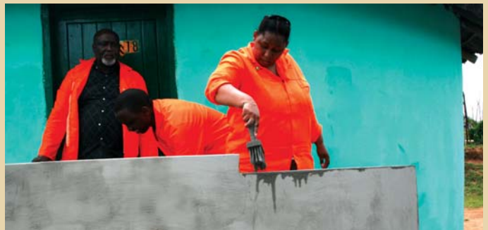
Deputy Minister Hendrietta Bogopane-Zulu applying cement wash on a ramp
