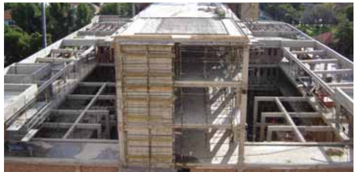
The second phase of the building
