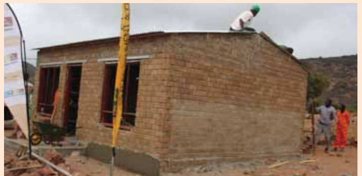
Doing final touches to the structure
