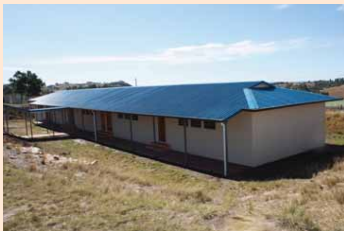
A block of classrooms at the new school
