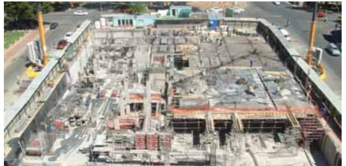
Foundation phase for the Bloemfontein Regional Office
