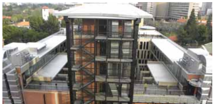
The completed structure
