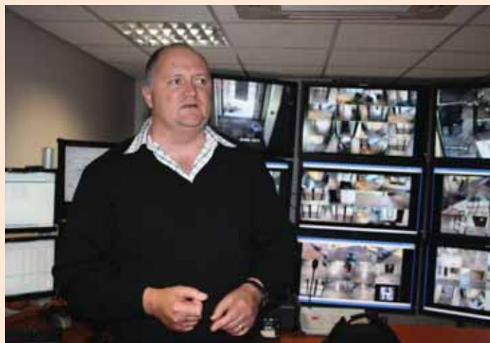
Mr Abrie Visser demonstrates in the Control Room
