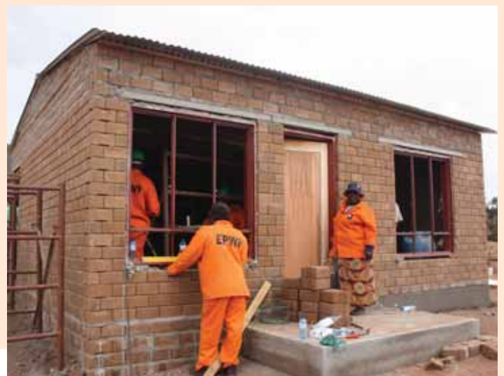
Doing final touches to the structure
