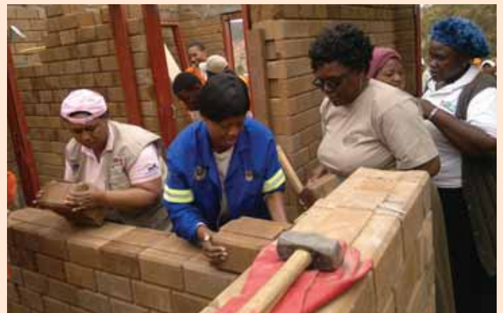
The house of the first beneficiary under construction
