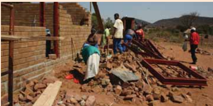
The house of the first beneficiary under construction
