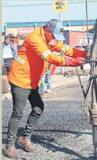
The Mpumalanga MEC for public works, roads and transport, Thulasizwe Thomo, takes part in pothole repairs during a road maintenance campaign at the Ermelo Long Distance Taxi Rank.
