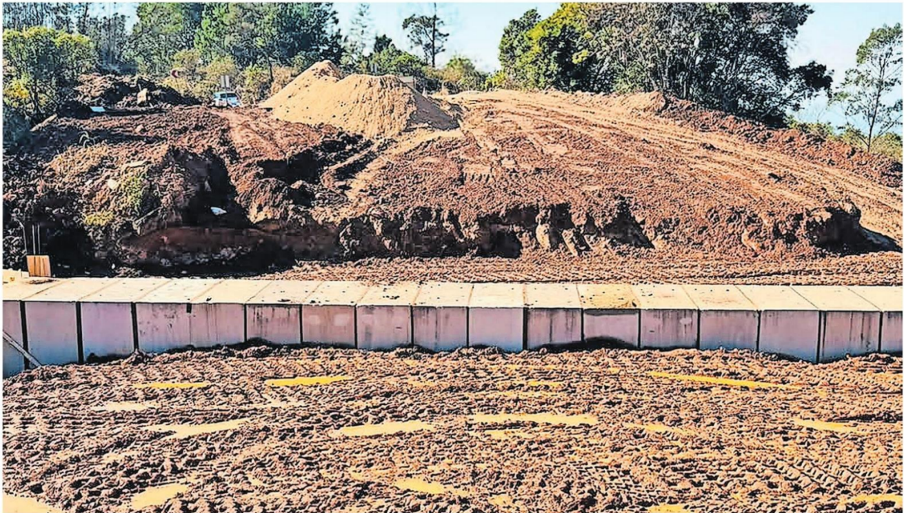
The progress of the road.
