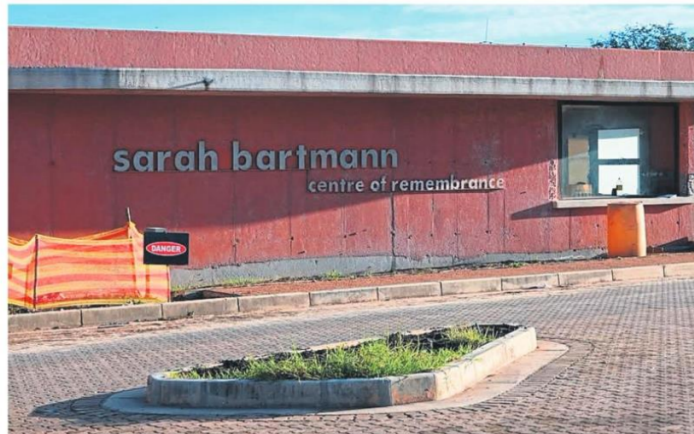
The construction of the Sarah Baartman Centre of Remembrance in Hankey was launched in 2014.
