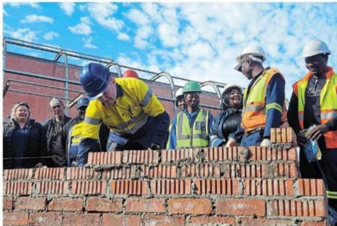
LAYING THE FOUNDATIONS: Public works & infrastructure minister Dean Macpherson, left, officially hands over the Sarah Baartman Centre of Remembrance site to contractors on Saturday. The restarted project's new completion date is October 2027. Picture: SIMTEMBILE NGIDI
