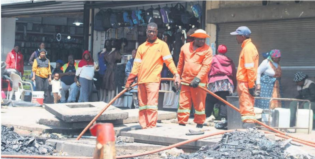
JRA workers clean a stormwater drain on 2nd Street.
