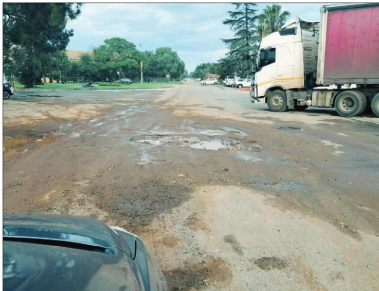
Huge potholes formed in Stilfontein roads after heavy traffic from the N12 was diverted through the town because of flooding. Photo: Tanya Pottas.
