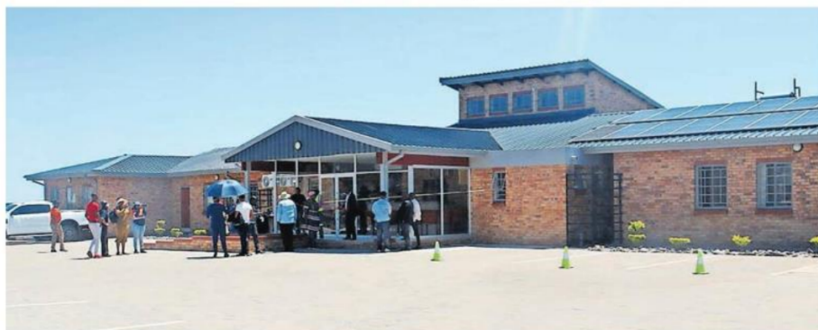
The newly built offices at Ga-Matsepe.
