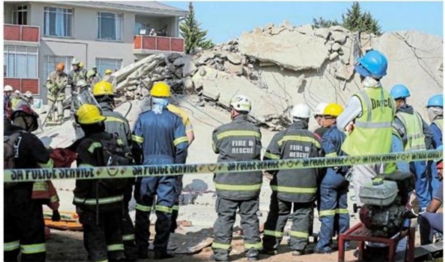
Rescue workers scour the rubble of the collapsed building in Victoria Street, George, in the Eastern Cape in May 2024. /Werner Hills
