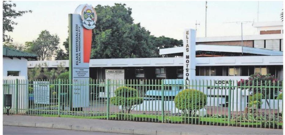
The Elias Motsoaledi Local Municipality offices.
