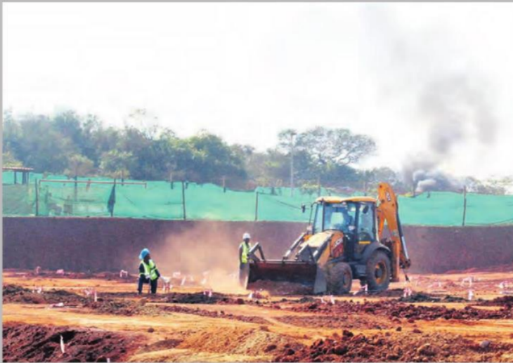
The construction site of the new orthotics and prosthetics centre at Ngwelezana Hospital
