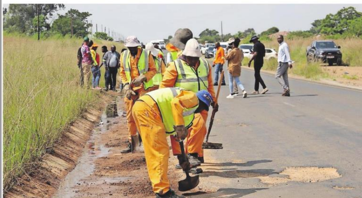
Road works in Moutse.
