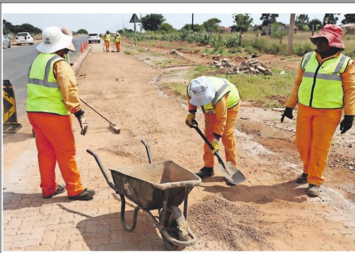
Workers busy on the rehabilitation project.
