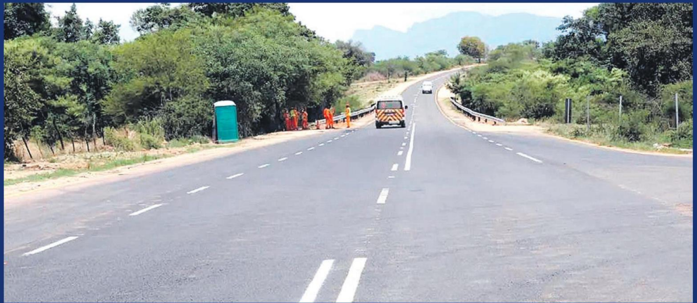
A smooth ride for motorists after the D21 was rehabilitated.
