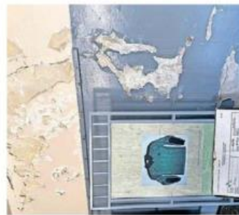
CONCERNS have been raised on social media about the alleged decaying and neglect of facilities at the Robben Island Museum. | LUKE AKAL
