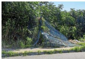
WASTED FUNDS: A close-up view of the damaged fence.
