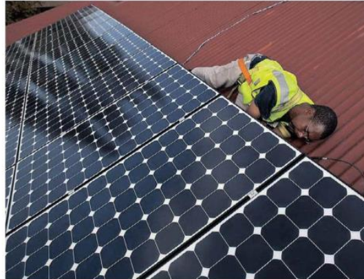
A WORKER installs solar panels on top of a roof. | SUPPLIED
