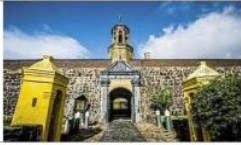
The Castle was built between 1666 and 1679, after the arrival of Dutchman Jan van Riebeeck.
