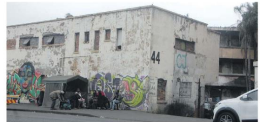
The Marikana building is where passersby, including women, are regularly mugged.
