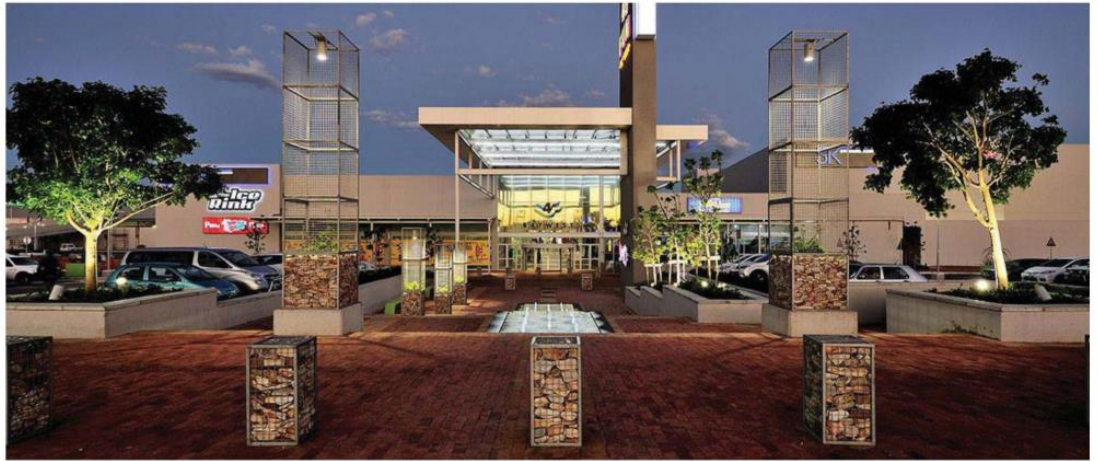
BAY WEST MALL in Gqeberha, the largest retail centre in the Eastern Cape, is being sold by Rebois in a public sale process, as part of the company's business rescue. | FILE
