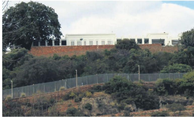
The estate incorporates 28 properties, including Mahlamba Ndlopfu, the official Pretoria home of President Cyril Ramaphosa, 15 tennis courts, a 9-hole presidential golf course and a helipad. Photo: Shaun Sproule
