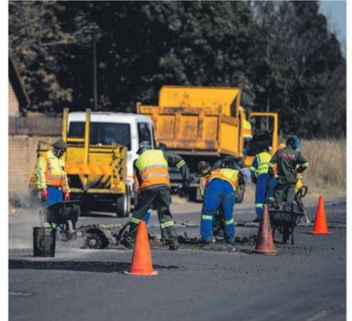
Workers repair the deteriorated roads in Ermelo. Photo | Wayne van der Walt
