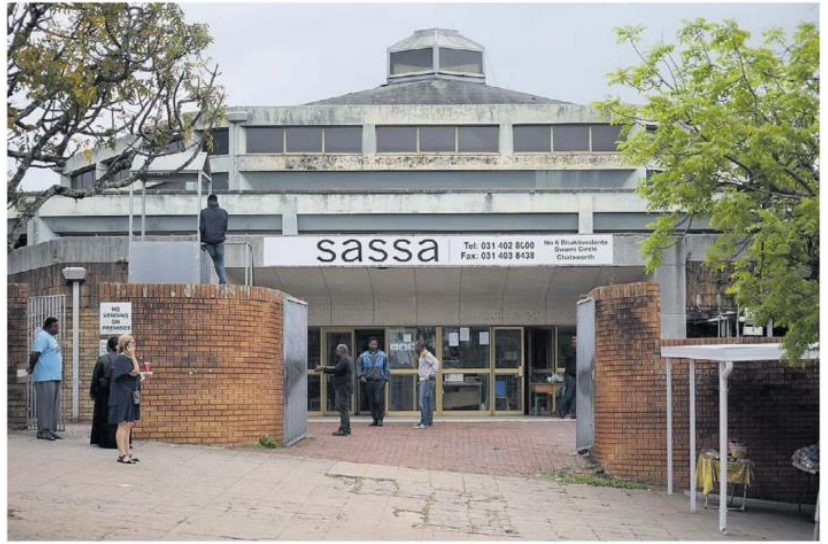
NOTICES were issued to the Department of Health, Department of Home Affairs and the South African Social Security Agency (Sassa) situated on Bhaktivedanta Swami Circle in Chatsworth, to vacate the premises until the building has been certified structurally safe for use by an engineer. | KHAYA NGWENYA
