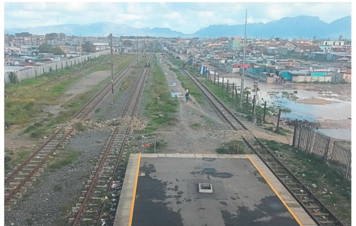
Railway tracks in the central line have been severely vandalised and in some instances people have moved on to the tracks.
