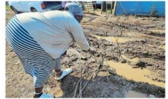
DEADLY THREAT: Nolitha Gadlela points out exposed electricity cables
