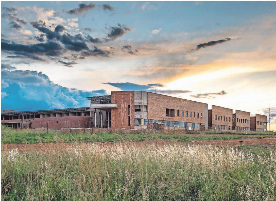
The Middelburg District Hospital is fast becoming a R1.8 billion white elephant. PHOTO: Enza Construction.
