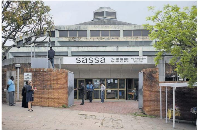
NOTICES were issued to the Department of Health, Department of Home Affairs and the South African Social Security Agency (Sassa) situated on Bhaktivedanta Swami Circle in Chatsworth, to vacate the premises until the building has been certified structurally safe for use by an engineer. | KHAYA NGWENYA
