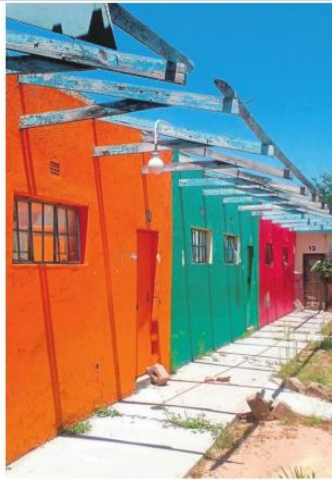
The roof at Makoko Primary was blown away after a storm years ago and has not yet been fixed.
