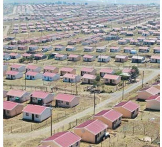
The Nquthu Phase 3 Housing Project.
